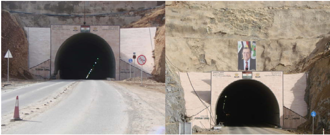
Back face ( Seetak area )
